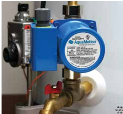
AquaMotionHot Two Dedicated Return-line Installation
