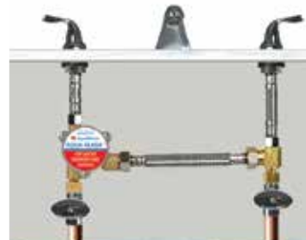
Flash Valve Installed
